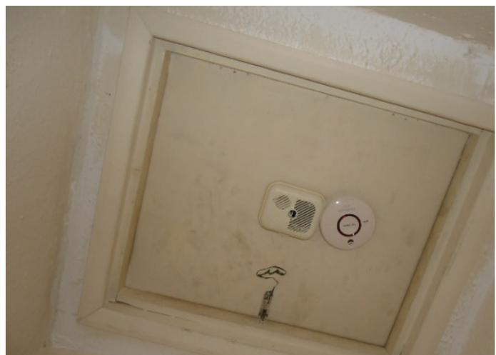
Loft hatch of unknown fire resistance not secured.
