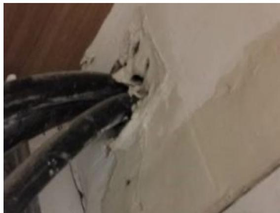
Poor stopping of gaps around cables.
